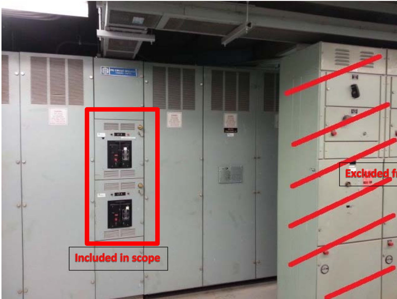
Figure 5 - 1960's Digester East Drawout Air Circuit Breakers
