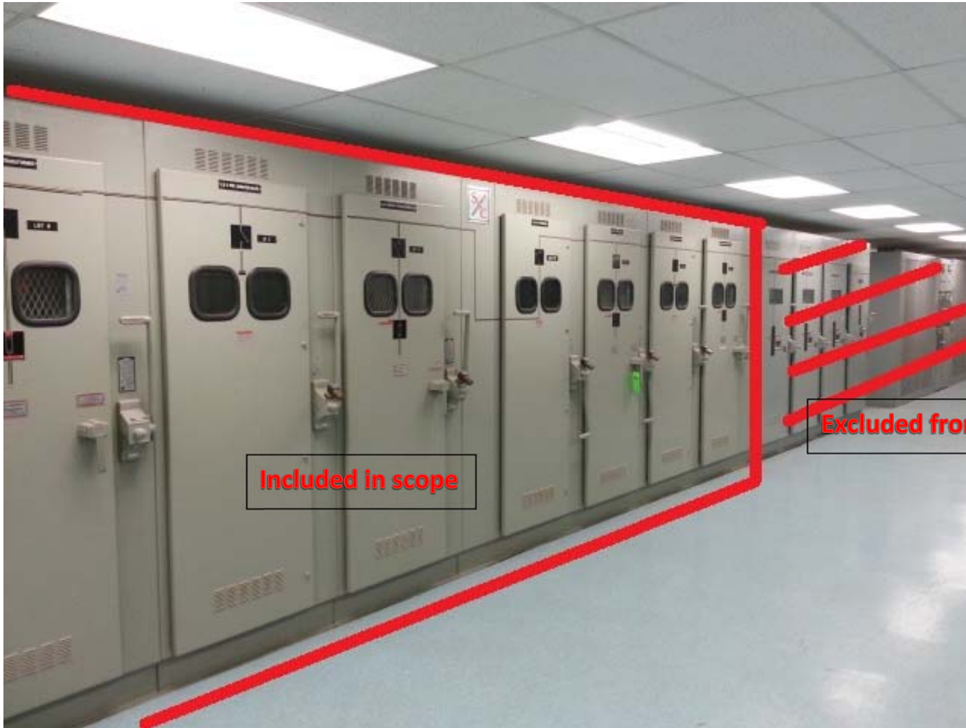
Figure 2 – 1960's Secondary Clarifiers Non-Drawout Disconnect Switches
